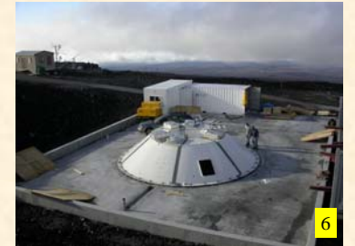
6 Hexapod supporting cone completion November 5 2004
