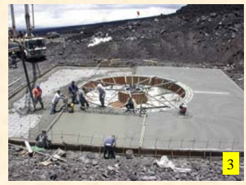
3 Concrete pouring May 15 2004
