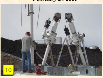
10 Hexapod jackscrew installation December 1 2004
