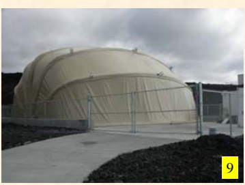
9 Shelter finished November 30 2004
