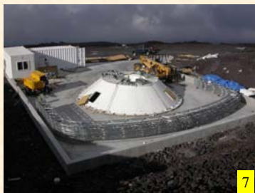
7 Shelter trusses assembly November 11 2004
