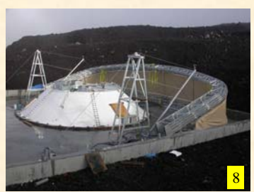
8 Partly completed shelter November 11 2004
