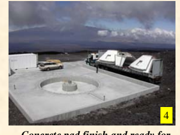
4 Concrete pad finish and ready for hexapod supporting cone installation October 17 2004
