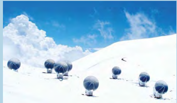
Figure -- Submillimeter Array (SMA) at the 4100m summit of Mauna Kea, Hawaii. The radio telescope combines eight 6-meter diameter antennas to carry out observations at submillimeter wavelengths at the highest spatial resolution in the world.
